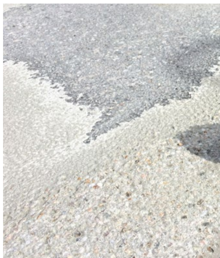
The remnants of a 10mm overlay after three passes with the HTC Ravager™
