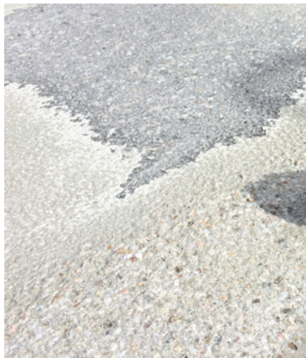
The remnants of a 10 mm overlay after three passes with the HTC Ravager™
